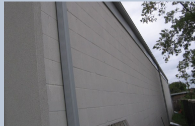
Figure B106 -Painted Concrete Block
