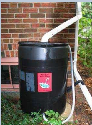
Figure D3 -Typical rain water barrel
