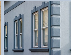
Figure B108 -Stucco (synthetic or natural)
